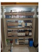
A relay logic circuit is an electrical network consisting of lines. The output is controlled by a combination of input or output conditions, such as input switches and control relays. The conditions that represent the inputs are connected in series, parallel, or series-parallel to obtain the logic required to drive the output.
